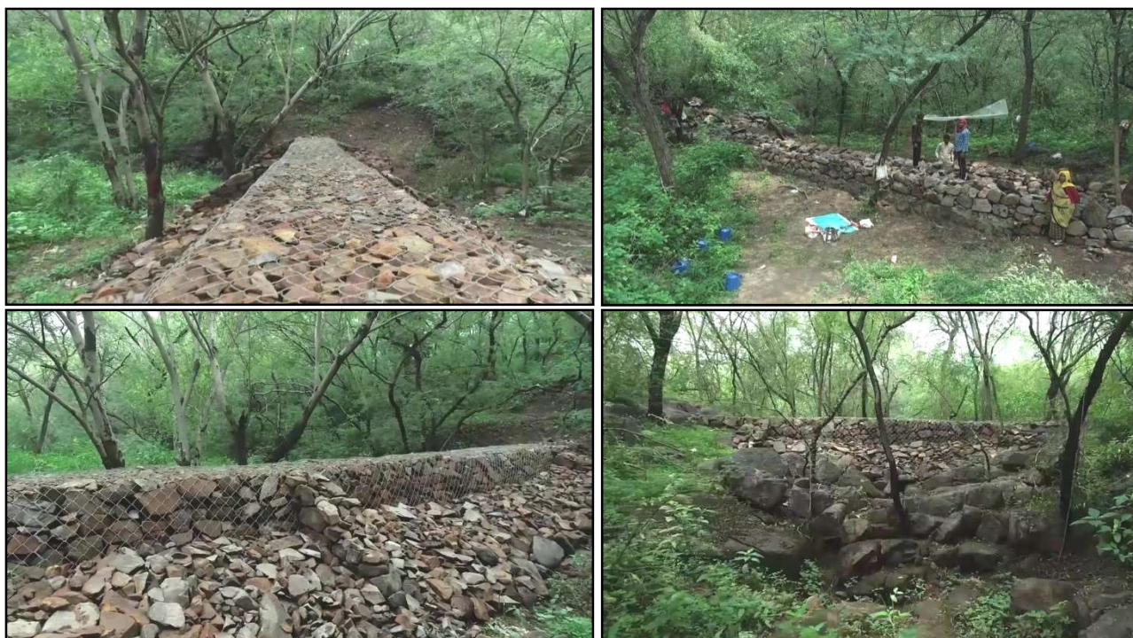
Figure: Creation of Checkdams in Asola Bhatti by Department of Forest and Wildlife, GNCTD
